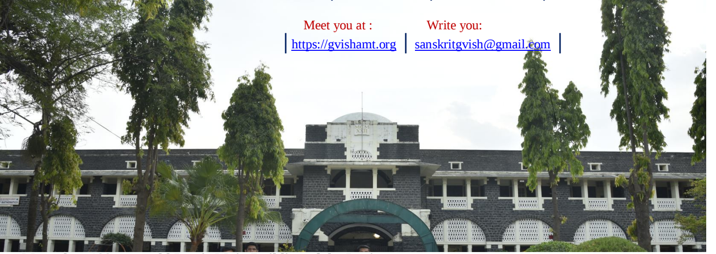
More than 100 years old Iconic Main Building of the Institute
