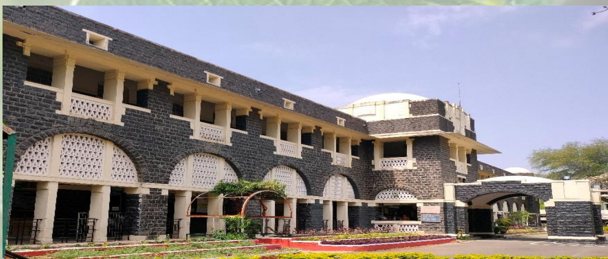
Iconic Heritage Building of The Institute
